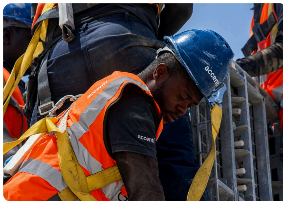
— Work at height with full-body harness and secured lanyards.
